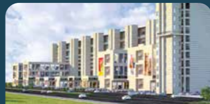
Mohali Citi Centre - 3 10 Acres Commercial Project F-Block Aerocity, Mohali
