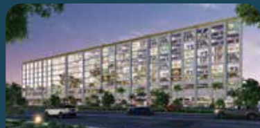
Mohali Citi Centre - 2 4 Acres Commercial Project F-Block Aerocity-Mohali
