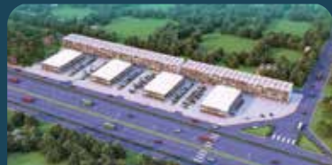
Mohali Citi Centre - 1 7 Acres Commercial Project F-Block Aerocity-Mohali
